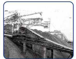
Selected coal was transferred to the storage facility via this conveyor belt, where it was kept before being loaded onto coal-carrying ships. The braces of the conveyor belt survive today.
